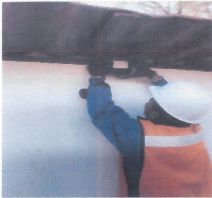
INSTALACION DE LUMINARIO LED IPO SUBURBANO 45W, 2470 LM
