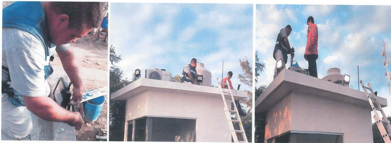
COLOCACION DE REFLECTOR LED FLOOD LIGHT 100W-6500K-100-265V-SMD
